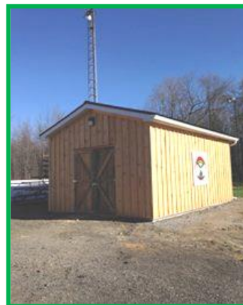
Photo: New Storage Building
